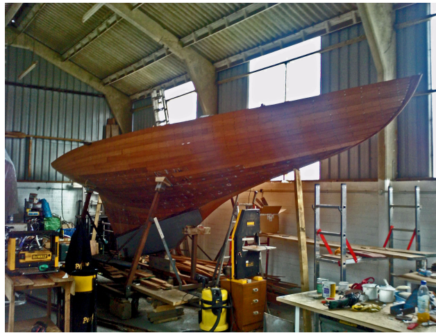
The top sides continued to full replacement of boards
